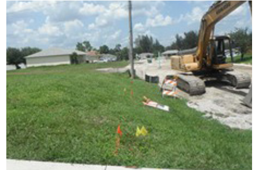
Flagged Utilities in ROW
