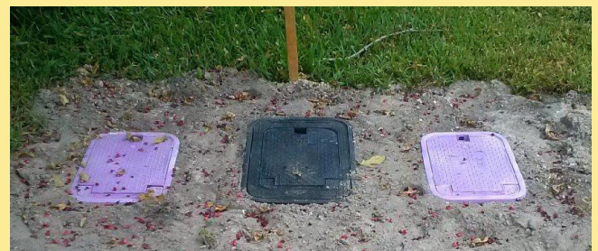
Water and Irrigation Meter Boxes
