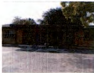
Area 7 – Residential Deterioration
