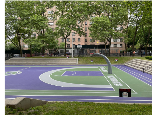
New York City's cloudburst infrastructure.
